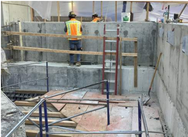
Progress at the Future Air Intake
