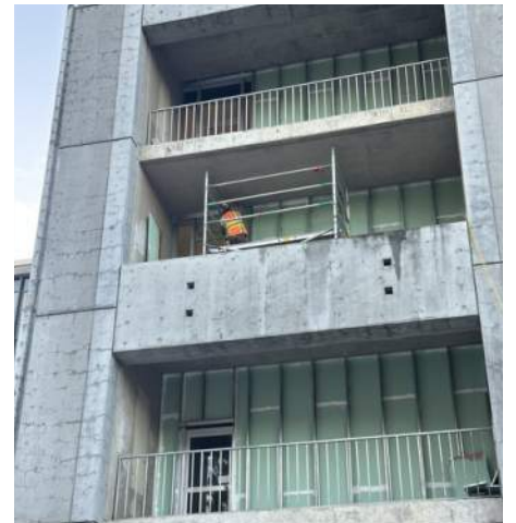
Protection Wall at the Existing Air Intake and Metal Stud Framing Installation at Latimer Hall
