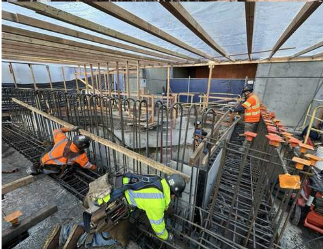
Progress of the Future Air Intake
