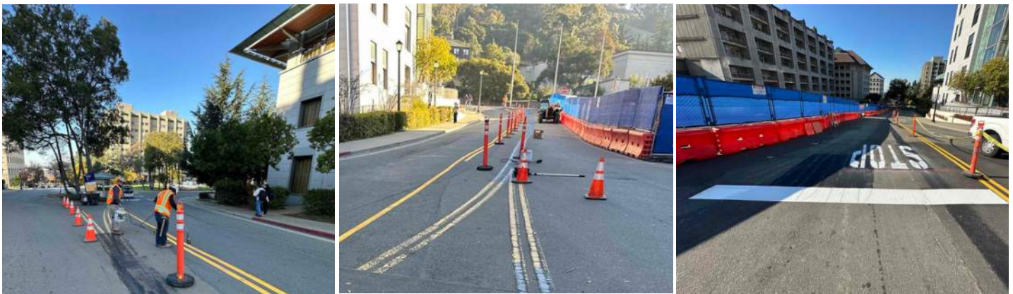
Progress Photos of Restriping at University Drive/Gayley Road
