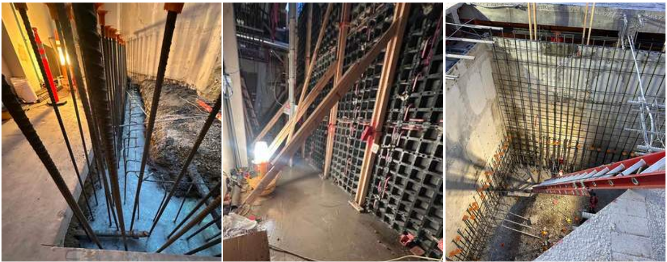
Progress Photos of Physics Space B18 / Future Air Intake
