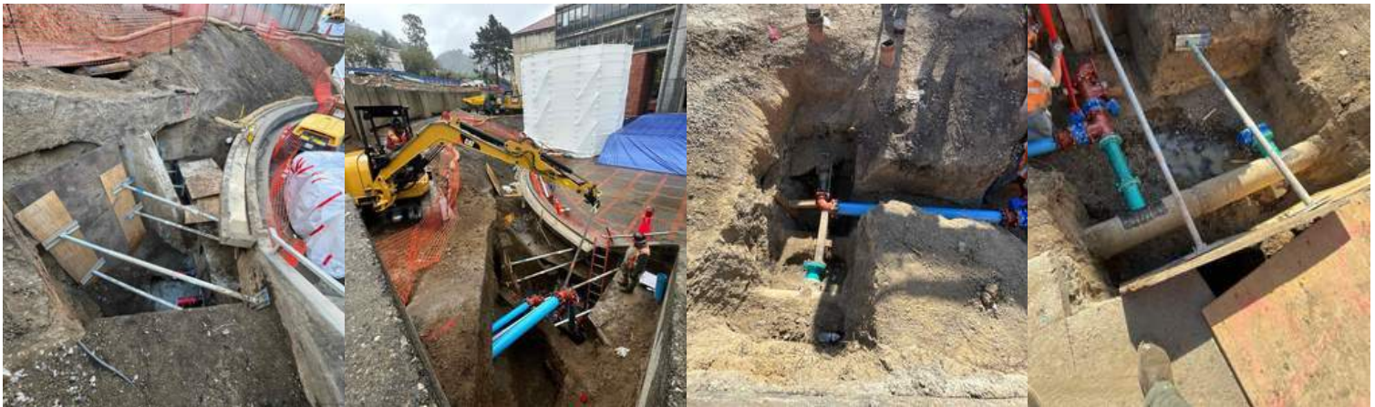
Progress Photos of Site Utility Shutdowns and Relocations
