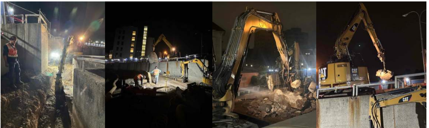
Site Trenching and Sidewalk Demolition
