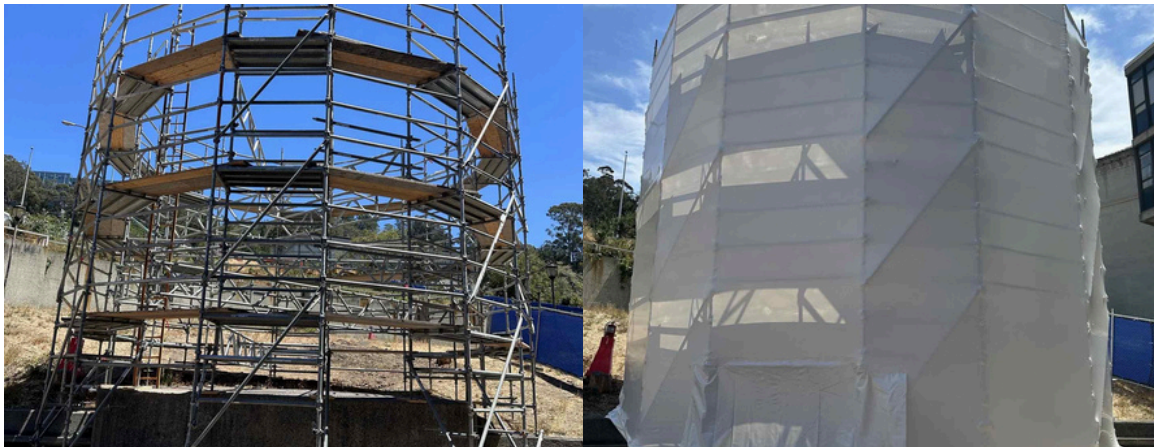
Latimer Hall Air Intake Before and After Wrapping Scaffolding Enclosure
