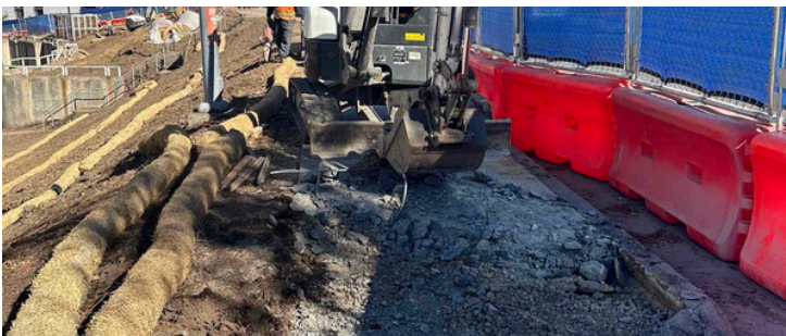
Sidewalk Removal at Gayley Road
