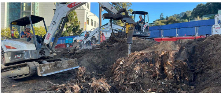
Tree Stump Demolition Near Gayley Road
