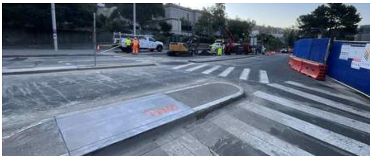
Potholing at Gayley Road
