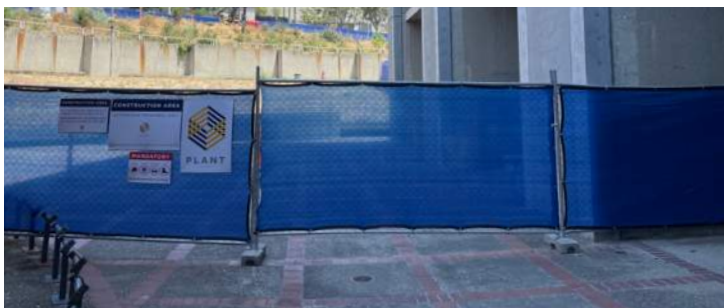
Perimeter fencing completed with signage
