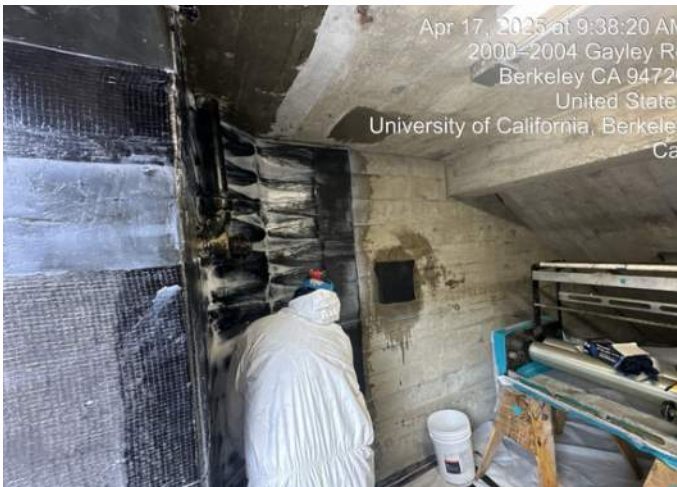
Applying FRP Layers at the New Lewis Hall Opening
