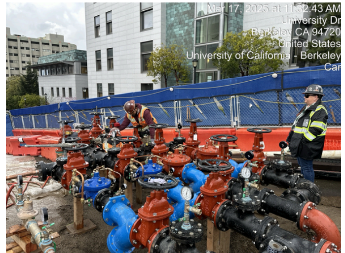
Newly Installed Pressure Reducing Valves
