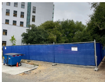
Fencing at laydown area 2 north east of Latimer Hall.
